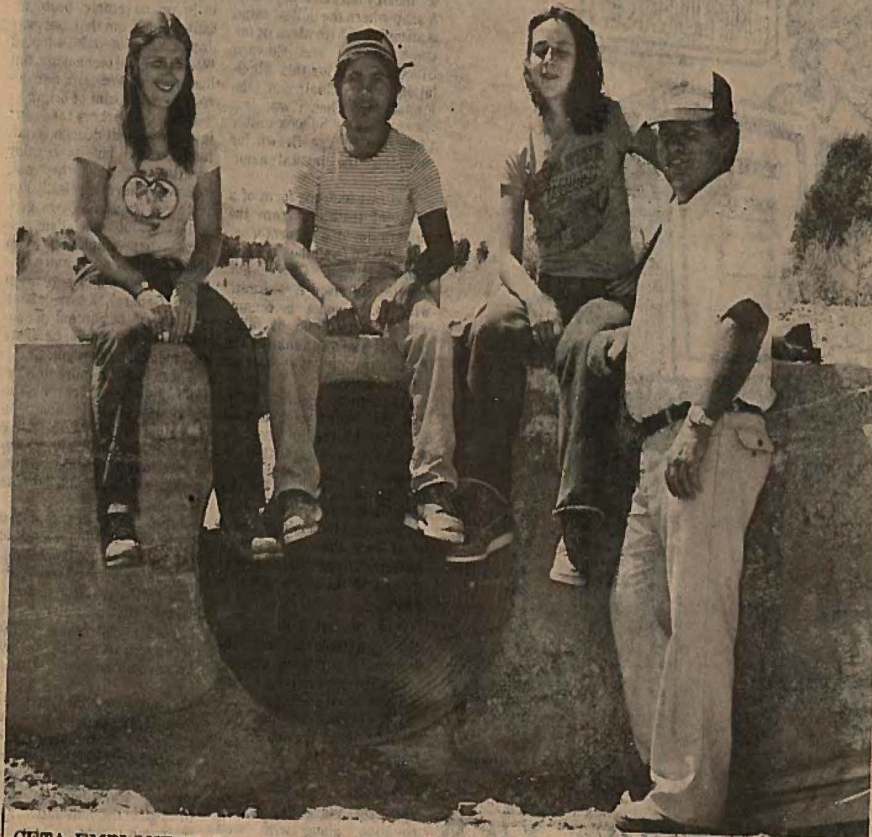
CETA EMPLOYEES, from left, Jill Greening, Leman Temoke and Kim Errecart along with Louis Horton are shown at a culvert recently installed behind Northern Nevada Community College. Horton is a supervisor of the project completed by CETA employees. Additional pictures of college construction projects appear on the back page of today's Free Press.
