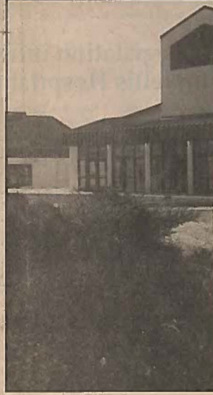
Great Basin College Theatre completed
