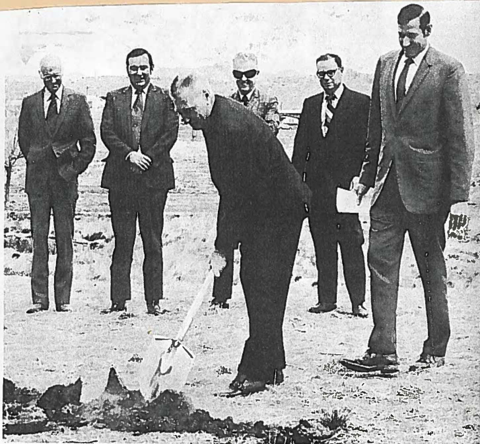
PAUL SAWYER WIELDS a shovel during Saturday groundbreaking ceremonies for the first building on the new Elko Community College campus, on the old municipal golf course near the National Guard Armory. Sawyer is shown here with (from left) Fred Harris, Mike Marfisi, Bill
