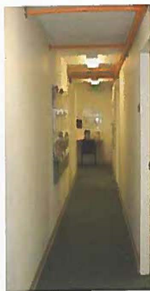
I'm heading down to the Security Offices. See the beautiful peach colored fire system.
